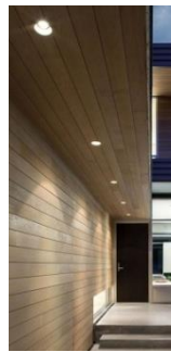
Downlights in the soffit to light the exterior pathway
