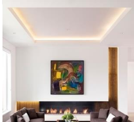
Illuminated ceiling coffer with linear LED
