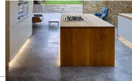
Bulkhead above kitchen island with linear LED around to uplight the ceiling. Downlights for task lighting. Linear LED concealed in the skirting board.
